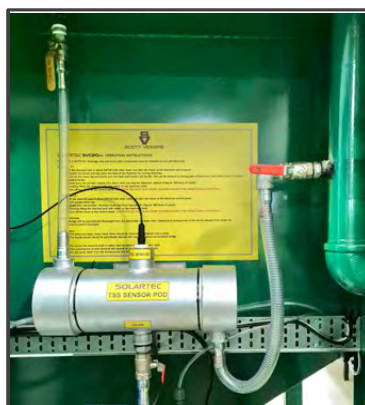
TSS SENSOR POD An alternative to the IBC Measuring Tank
