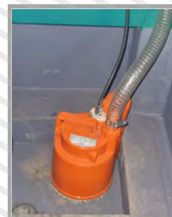
Water Transfer Pump Exuded water is transferred back into the system for suspended solids removal
